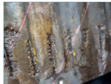
Corroded Reinforcement causing concrete spalling in the external launder wall of the tank
