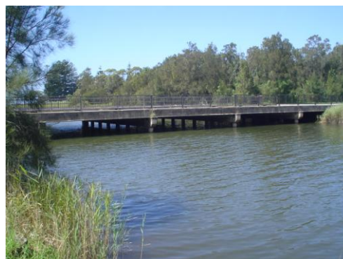
Fairy Creek Bridge
