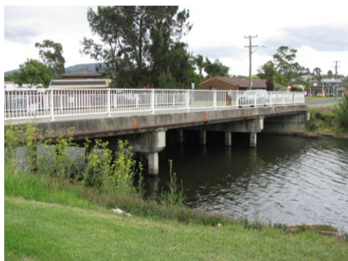
Brooks Creek Bridge
