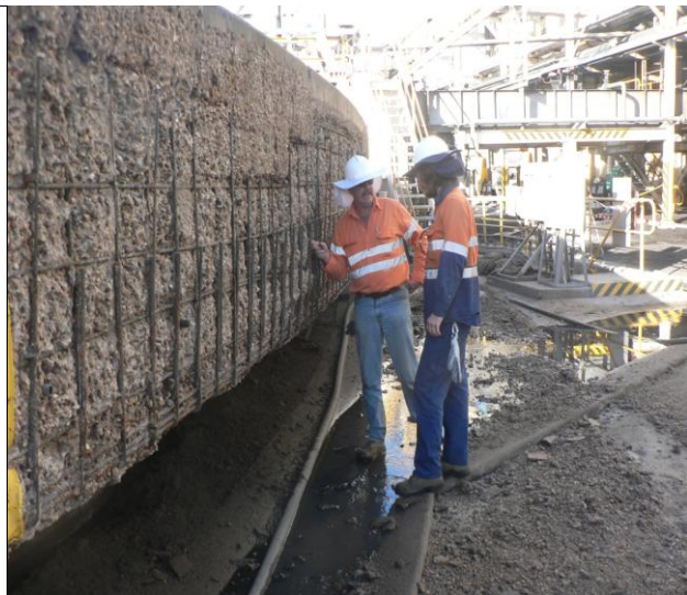
Launder wall after hydro-demolition has removed the delaminated and spalling concrete.
